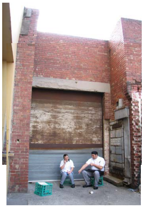
6 Radisson restaurant staff take breaks in the alley. Mazda roller door is used occasionally - they ask the restaurant staff to move their cars if necessary. This fire door cannot be blocked.
