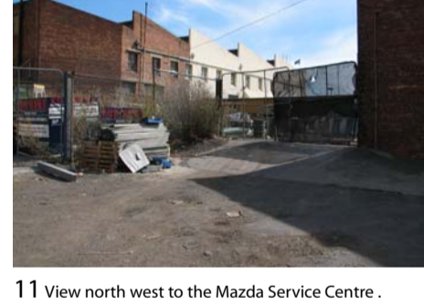
11 View north west to the Mazda Service Centre.
