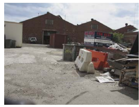
9 View north to the existing Rock Emporio building.
