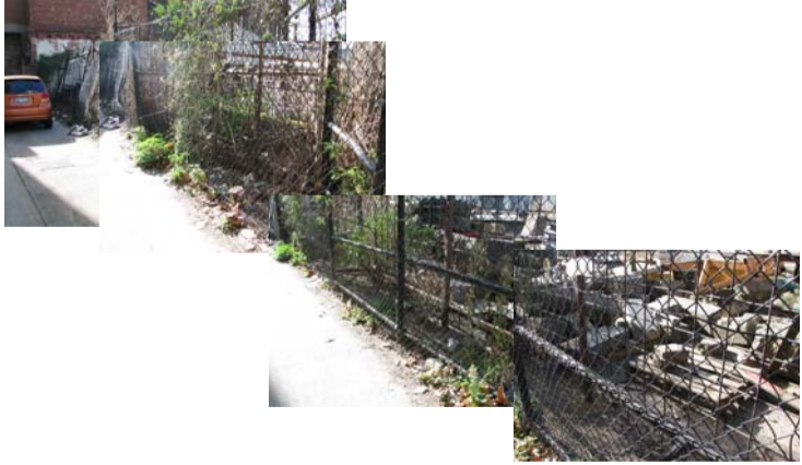
12 The fence has an old access gate and pedestrian walkway.
